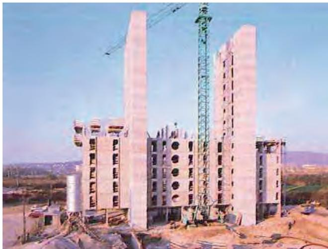
The continuity of the assembly is an essential feature of the system thanks to the sufficient width of the base of the columns. Even with a modest additional seasoning of the concrete in situ, the columns are able to withstand the weight of several floors. The result is a rapid progress of work. The structure was subjected to laboratory tests, through the realization of true joints, in order to verify the static behaviour in the most difficult operating conditions.
