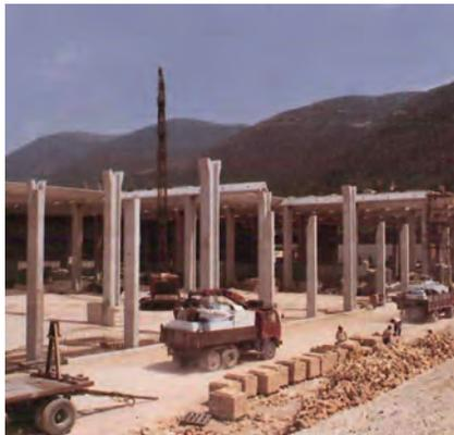
Roofing elements (tegoli) prestressed and manufactured on site
