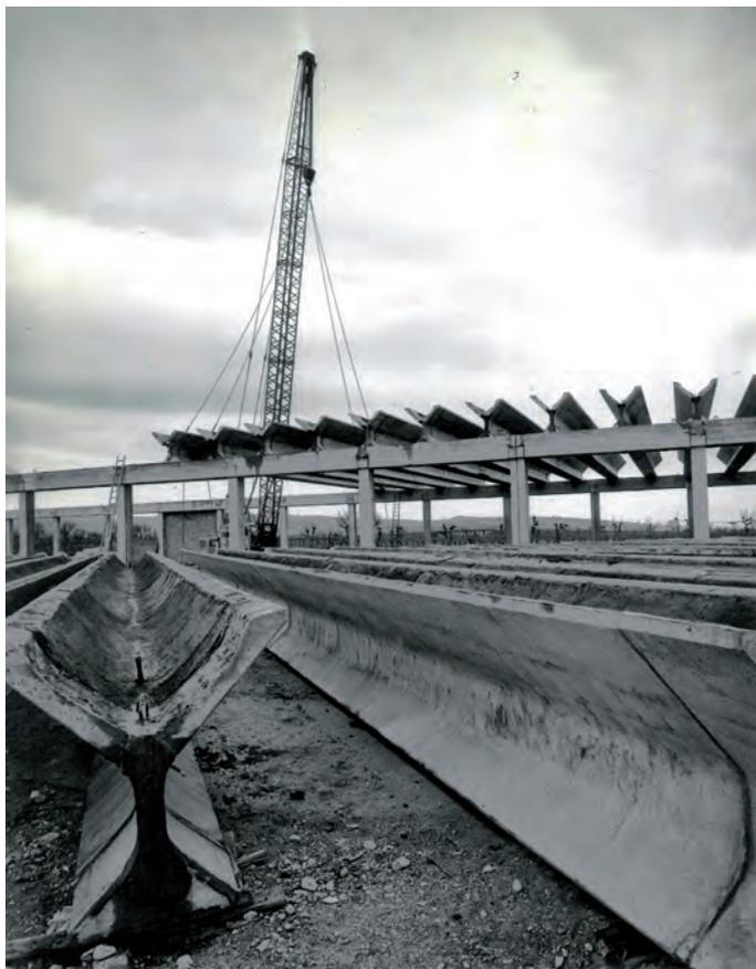
Roof elements (tegoli) precast in site, prestressed and post stretched
