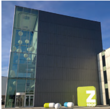
ZAMBON S.P.A. Z BUILDING (Vicenza)
